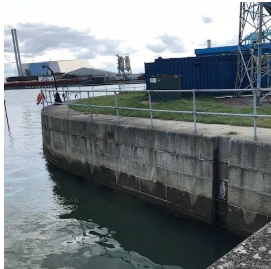
Fig 9: The wrought granite of the Pier Head, scheduled to be salvaged
