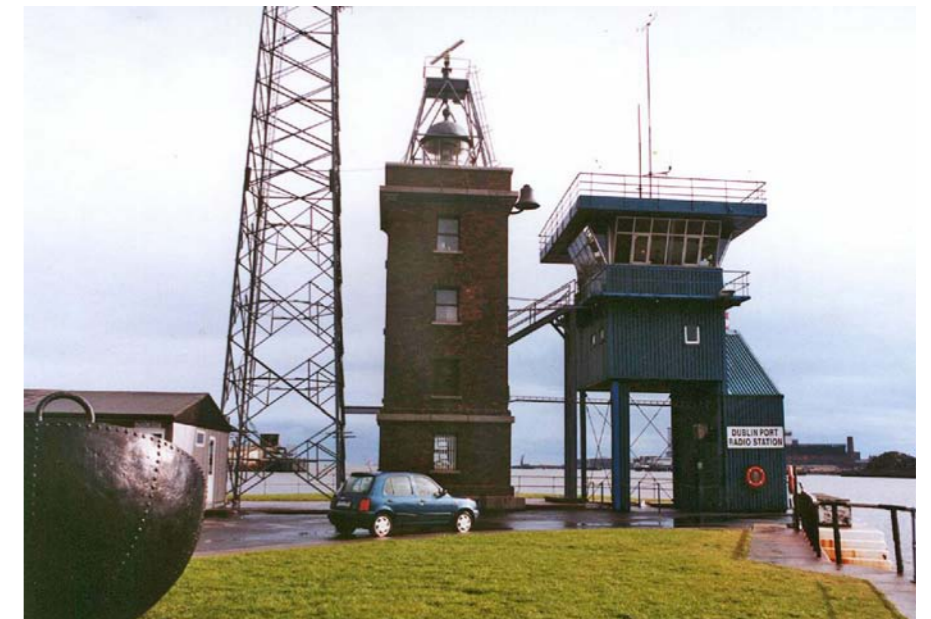
Fig 4: The Breakwater (or Alexandra Lighthouse) in the mid 1980's
